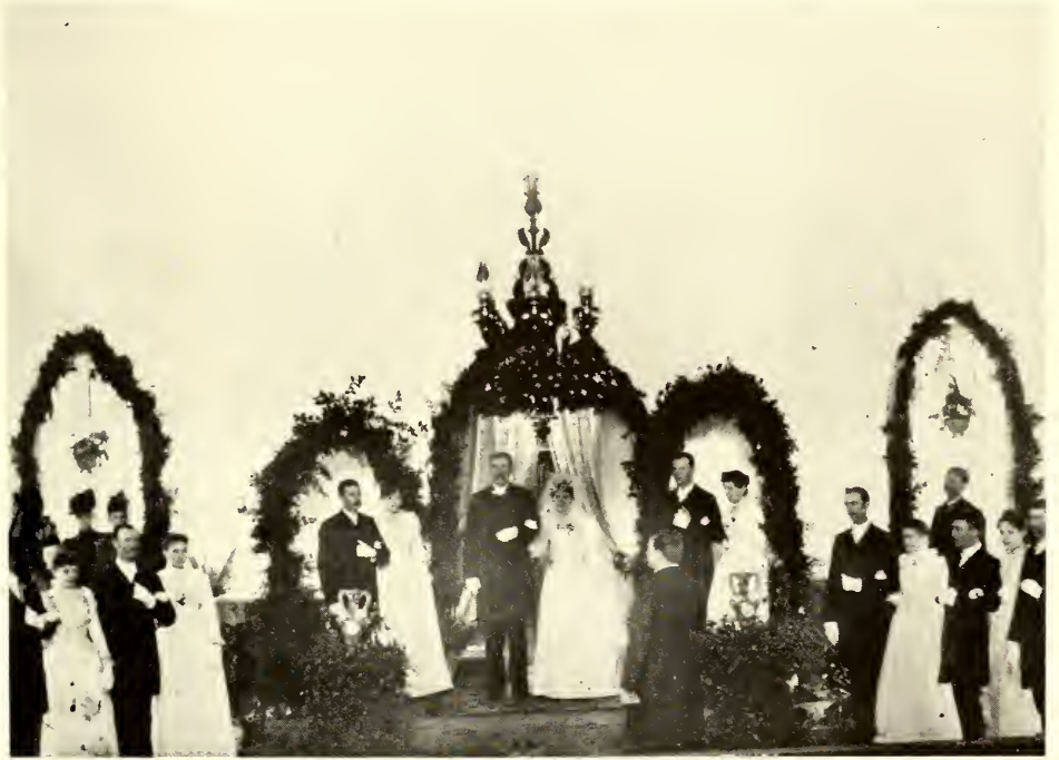
Auditorium of the second church before it was completely finished on Christmas Eve, 1889 at wedding of William Hackett Blanton and Della Hamrick, parents of Mrs. Pansy Blanton Fetzer. The church was overflowing for the elaborate wedding, first to take place in the church and at which Rev. J. M. McManaway presided. A reception followed at the Commercial Hotel. Members of the wedding party were (not all pictured): Addie Lynch (Mrs. Will Dameron), Dora Hamrick (Mrs. W. H. Jennings), Ollie McBrayer (Mrs. S. S. Royster), Julia Wilson (Mrs. J. D. Andrews), Fannie Wray (Mrs. John Hudson), Hattie Kendrick, Kitty Andrews, Emma Suttle, Cleo Gardner (Mrs. Tom Robinson), Hattie Lattimore (Mrs. W. B. Nix); H. Decatur Wilson, W. C. Corbett, S. S. Royster, J. F. Ware, C. C. Gidney, Hill Blanton, James Wilson, Dr. J. A. Harrill, W. B. Wray, B. E. Hamrick.
